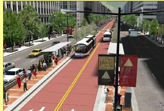
BRT vehicles can run either in mixed traffic or in a separate right-of-way. Above: an artist's rendering of the K Street Busway in Washington, DC.
